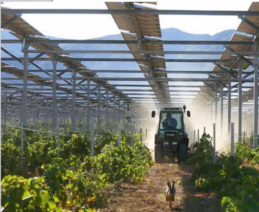
System with high mounting structure and continuous rows of PV modules.
